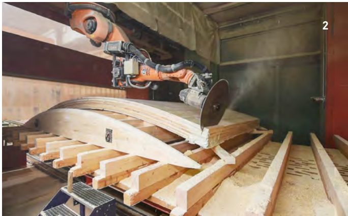
1 Fuggerei NEXT500 Pavillon, Augsburg; © Sandra Sitzmann / 2 LENO®-Element, Roboterabbund
