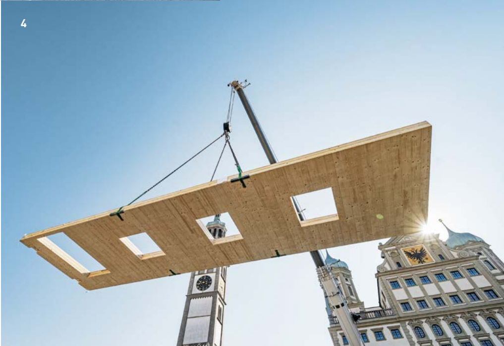
2 KUKA CNC robot © Sandra Sitzmann/ZÜBLIN Timber / 3 Serial elements on the construction site © Sandra Sitzmann/ZÜBLIN Timber / 4 Fuggerei NEXT500 pavilion, Augsburg (DE) © Eckhart Matthäus
